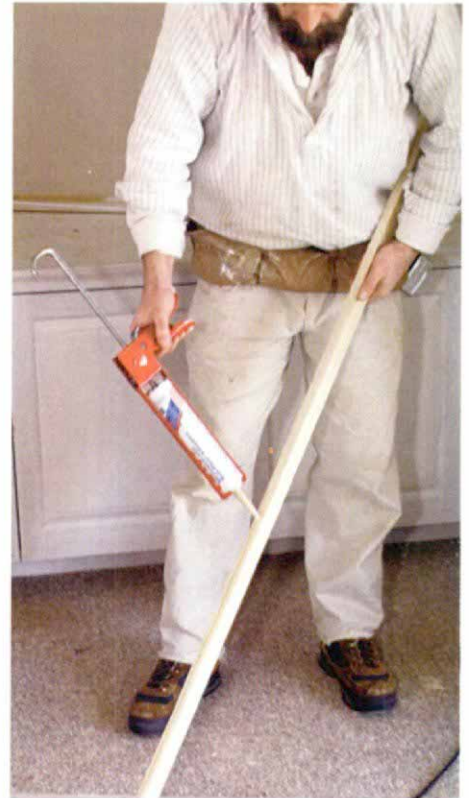
Face frames are glued to the walls. To help stabilize the sides of the shelf sections, the face-frame edges are coated with construction adhesive before being nailed to the shelf sides.
