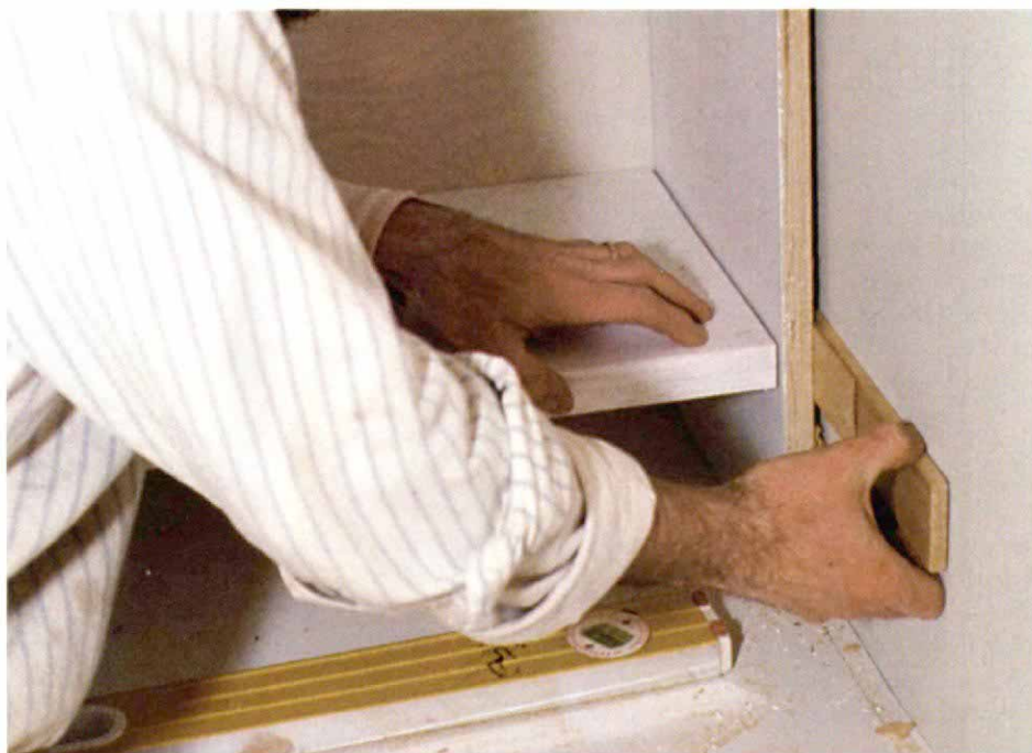
Scribing with a pencil. To scribe variations of less than \frac{1}{8} in., the author lets a pencil ride on the wall, its point recording the scribe line.
