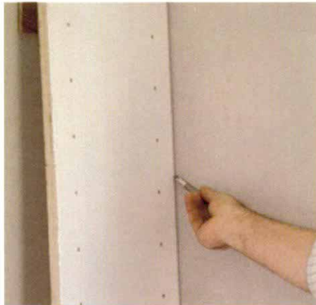
Scribing with a pencil. To scribe variations of less than \frac{1}{8} in., the author lets a pencil ride on the wall, its point recording the scribe line.
